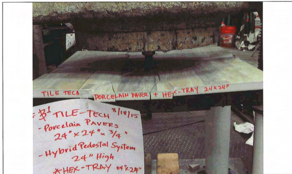
Photo No. 4: General view of Hex-Tray Sample Failure
