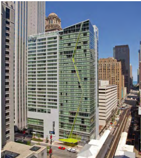
Above & Right : Wit Hotel - Chicago, IL Architect: Koo & Associates Application: Roof Deck - Pedestal Set Size & Color: 16" x 16" Stamp-Tech: Slate Black
